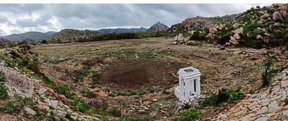
A dried up tank in Chitradurga; a tank work in progress inside the KSRP batallion in Hosapete. DH PHOTOS/BH SHIVAKUMAR
